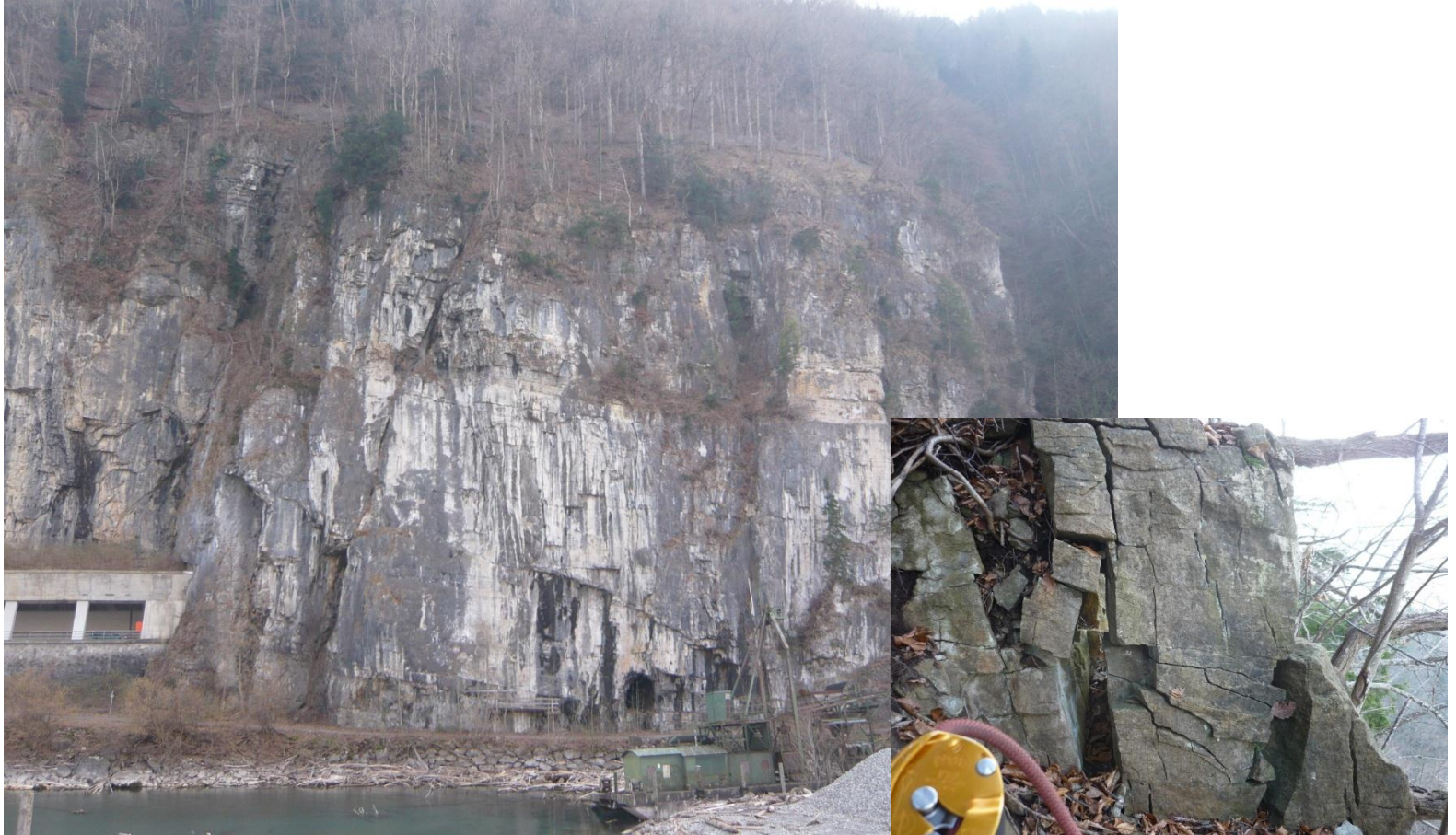
Weisswand West: Felsräumung (2013)
